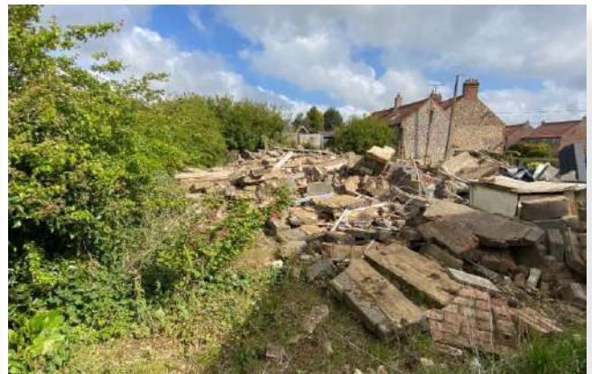
The site from the north east corner facing south west
